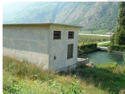
Station de pompage
