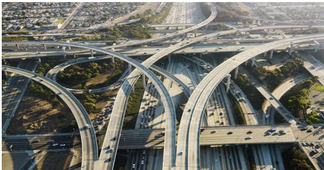
Fig 13: Echangeur autoroutier " los Angeles "
