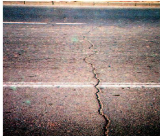
FIGURE 3. Fissuration transversale
